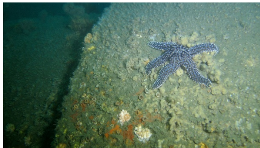
Sea Star on the Outfall Pipe
