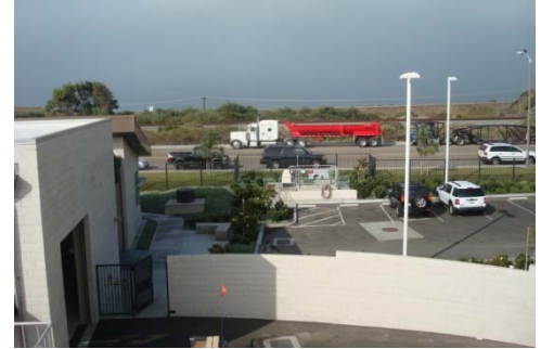
Figure P-2.1.002 View towards Ocean Outfall
