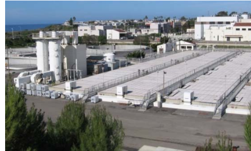
Figure P-1.3.003 Aeration Basins
