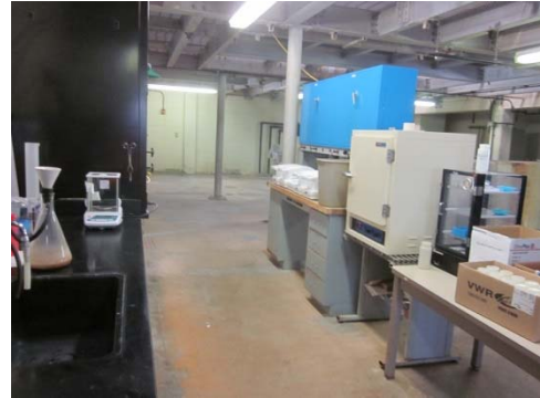
Figure P-5.3.010 Dryer Laboratory
