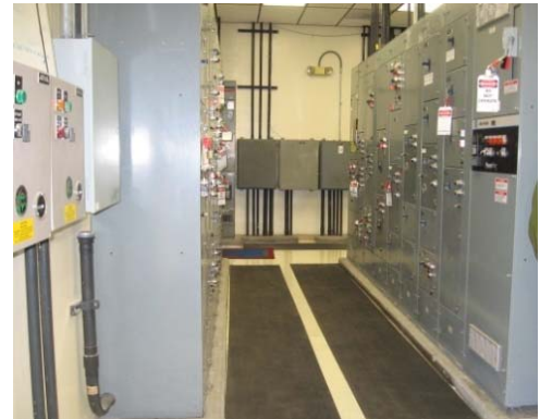
Figure P-3.3.001 Power Building MCC
