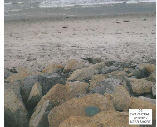
Figure P-2.1.006 Outfall near Shore
