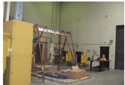
Figure P-4.1.008 Future Co-Gen Engine 5 location
