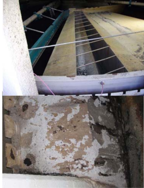
Figure P-3.1.001 DAFT Collector and Launder
