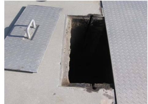
Figure P-1.1.006b Grit Influent Tank No. 3
