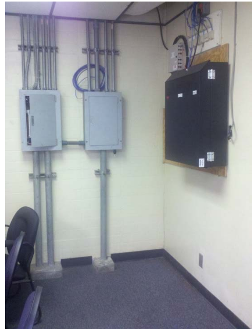
Figure S-5.3.003 Electrical Equipment
