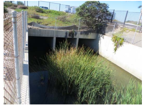
Figure P-5.2.028a Flood Channel within the Plant
