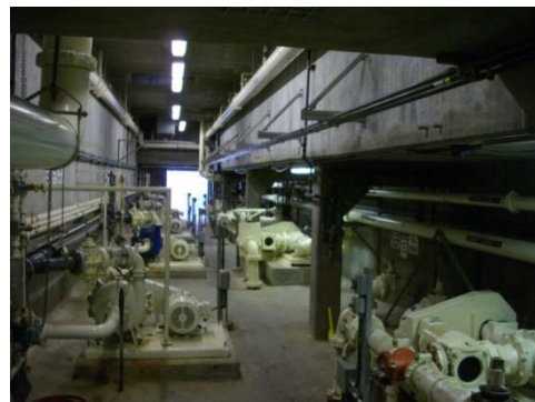
Figure P-1.2.002 Primary Sludge Pump Gallery
