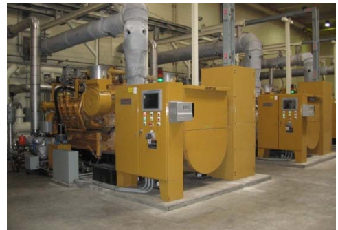
Figure P-4.1.005 Cogeneration Engine Nos. 1 and 2
