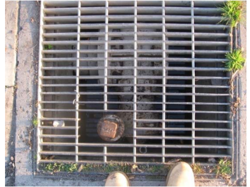
Figure P-5.2.015 Stormdrain near DAF Pit
