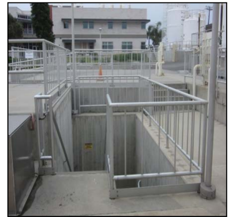
Figure P-5.2.028b Middle Primary Pump Gallery Entrance
