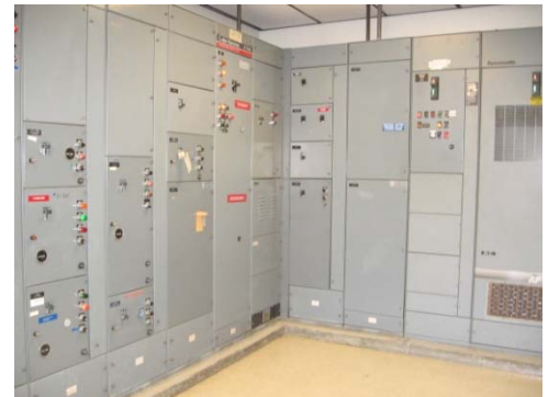
Figure P-1.4.002 Effluent Pump Station MCC Room
