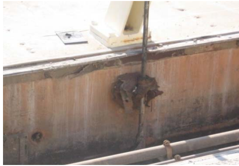
Figure P-1.2.006e Primary Influent Gate Guide Corrosion
