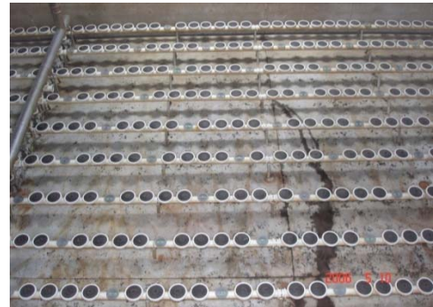
Figure P-1.3.005 Aeration Basin Diffusers
