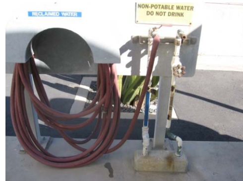
Figure P-5.2.017 Service Air/Washdown Station
