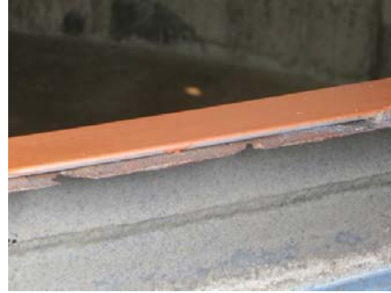
Figure S-8.2.013c Highly Corroded Skimmer Wear surface was rehabilitated by EWA Gen Services
