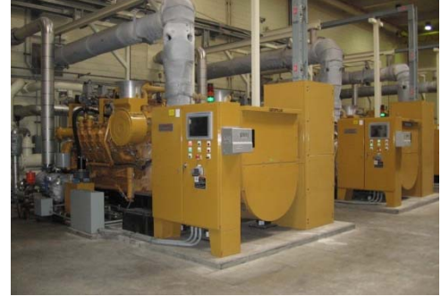
Figure P-4.1.007 Cogeneration Engine Nos. 1 and 2
