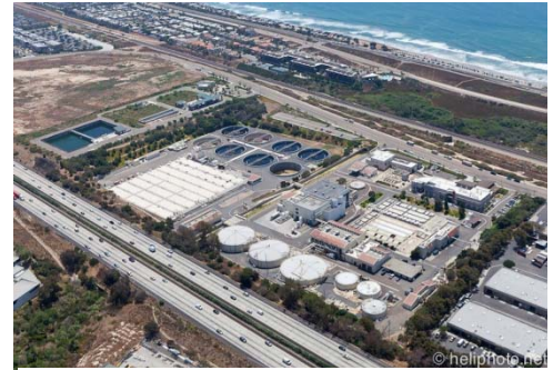
Figure P-5.1.004 EWPCF Aerial View
