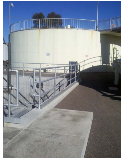
Figure P-3.2.007 Digester No. 1
