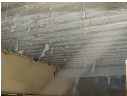
Figure S-8.3.013d Aluminum roof coating is failed in DAFT 1
