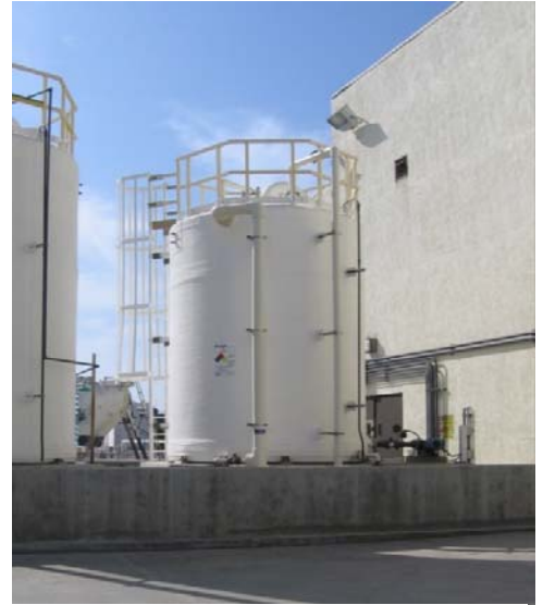
Figure P-3.3.017 Dewatering Polymer Storage Tank
