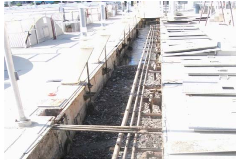
Figure P-1.2.006f Primary Influent Channel
