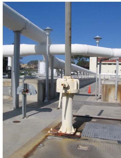
Figure P-1.2.004b Primary Effluent – Secondary Bypass Flow Control Gate
