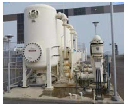
Figure S-8.2.013g The DAFT system is composed of many components EWA maintains
