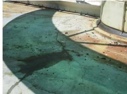
Figure P-1.3.013 Secondary Clarifier Cracking
