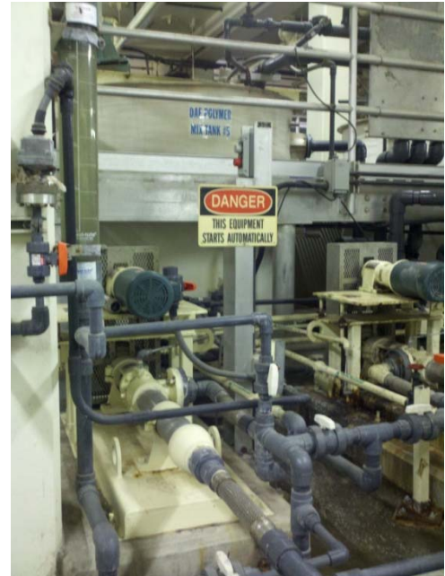
Figure P-3.1.004 DAF Polymer System
