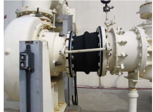
Figure P-3.2.013 Digester 6 Pump
