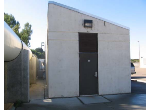
Figure P-5.2.021 SEEPS MCC Facility
