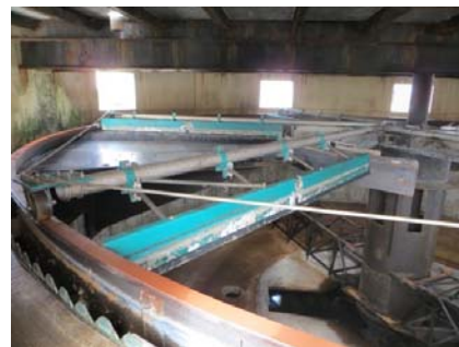
Figure S-8.2.013e Many mechanical and structural components require ongoing maintenance
