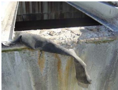
Figure P-1.2.006a PSB – Top of Wall Corrosion
