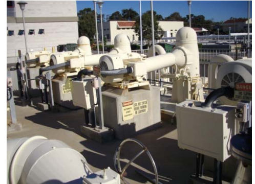
Figure P-1.4.001 Final Effluent Pumps
