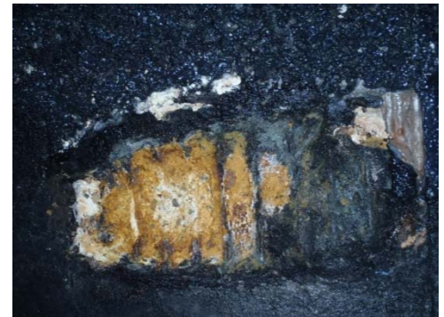
Figure P-1.2.009 Crown of PE Pipeline
