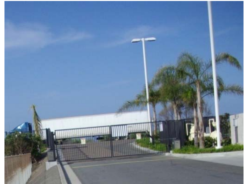
Figure P-5.2.012 Contractor's Entrance to Site
