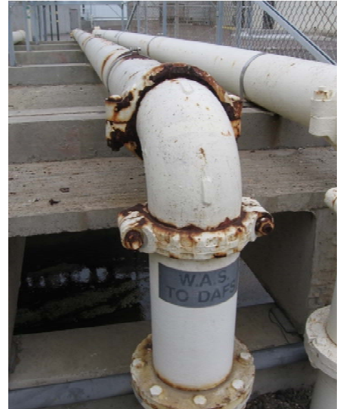
Figure P-1.3.010 WAS Pipeline
