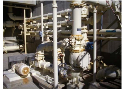
Figure P-3.1.003 TWAS Pump and Discharge Piping
