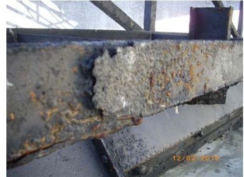
Figure P-1.3.007 Secondary Clarifier Nos. 5 and 6 Corrosion
