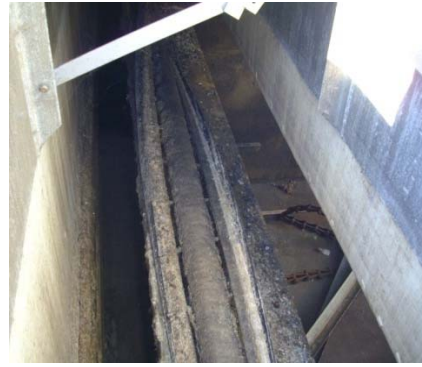
Figure P-1.2.006b PSB Helical Scum Skimmer
