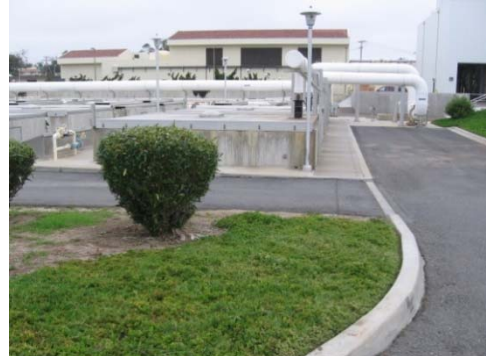
Figure P-1.2.003 Primary Effluent Channel
