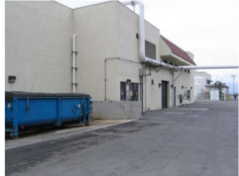
Figure P-5.1.001 Existing Headworks Facility
