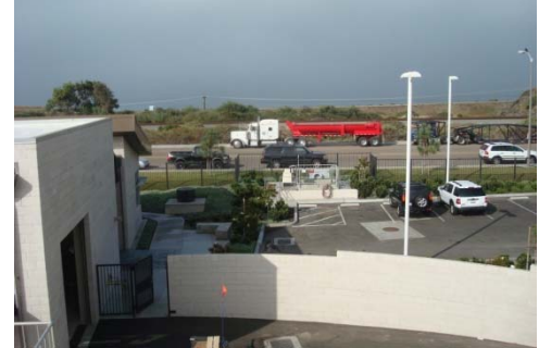
Figure P-2.1.004 View towards Ocean Outfall
