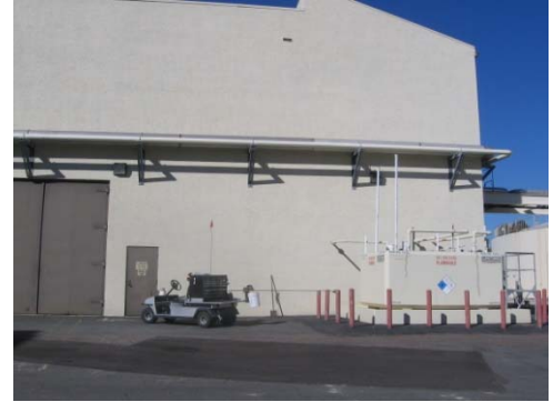
Figure P-4.1.009 Potential Location Identified for Future Co-Gen Engine
