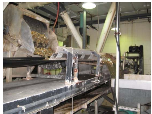
Figure P-1.1.005 Bar Screen Conveyor
