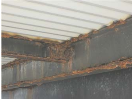
Figure S-8.2.013b Roof supports and hardware in DAFT 3 are corroded
