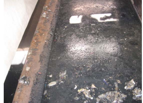
Figure P-1.1.006a Grit Tanks Effluent Channel
