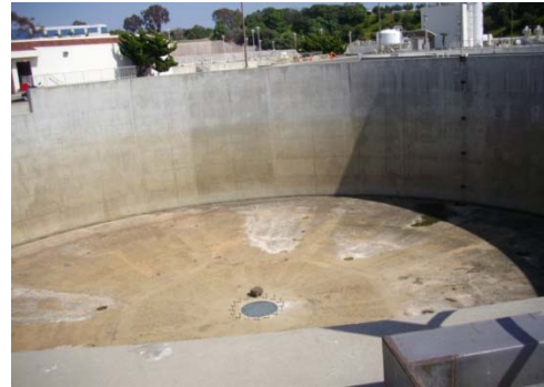
Figure P-1.3.008 Secondary Clarifier No. 7 Tank
