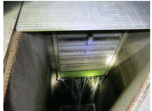
Figure P-1.3.014 Secondary Clarifier Effluent Gates
