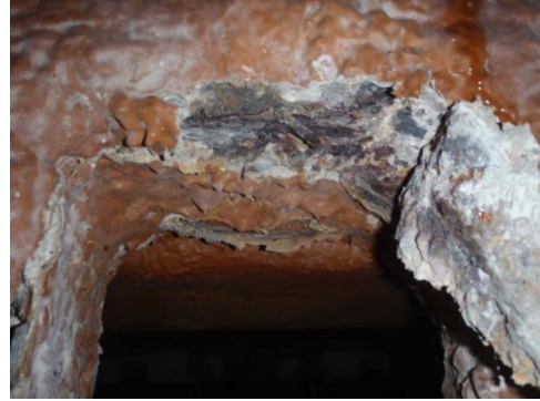
Figure P-1.2.006d PSB Previous Concrete Coated Over
