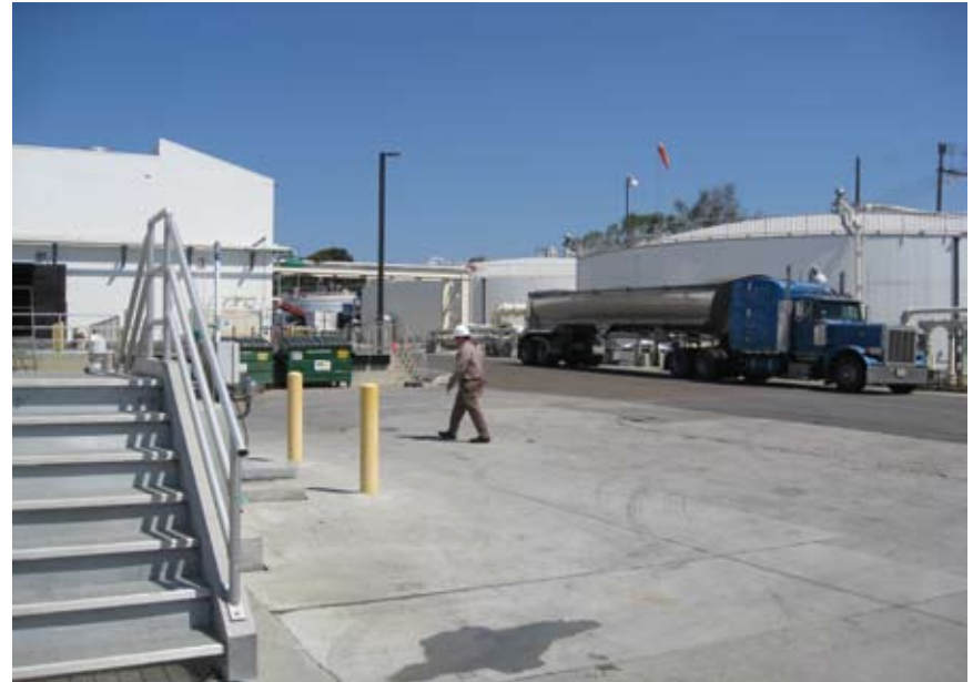
Solids Handling Systems Area Photo
