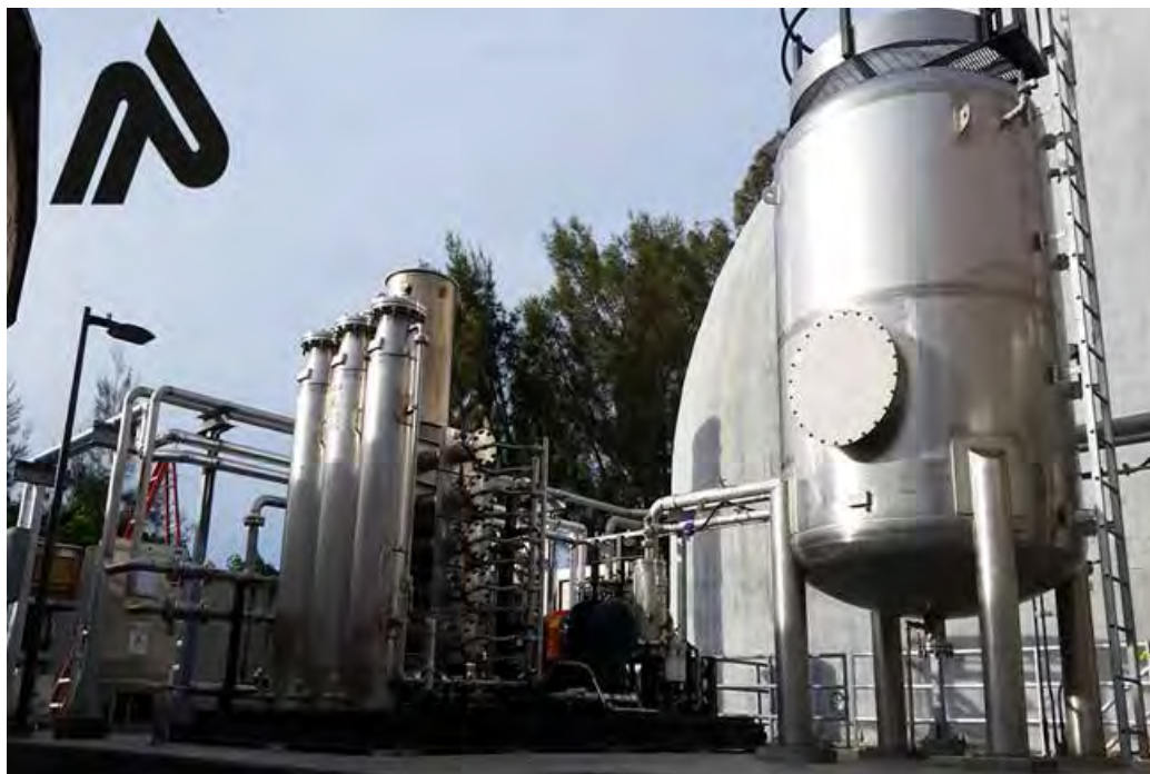
Figure 4-1. DG upgrading system at the San Mateo Wastewater Treatment Plant (California) using Unison's BioCNG system Includes \text{H}_2\text{S} removal, moisture removal, compression, siloxane removal, and membrane separation.
