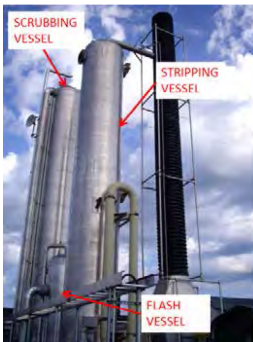
Figure 4-5. Greenlane Totara plus process vessels at Fair Oaks Dairy in Indiana
