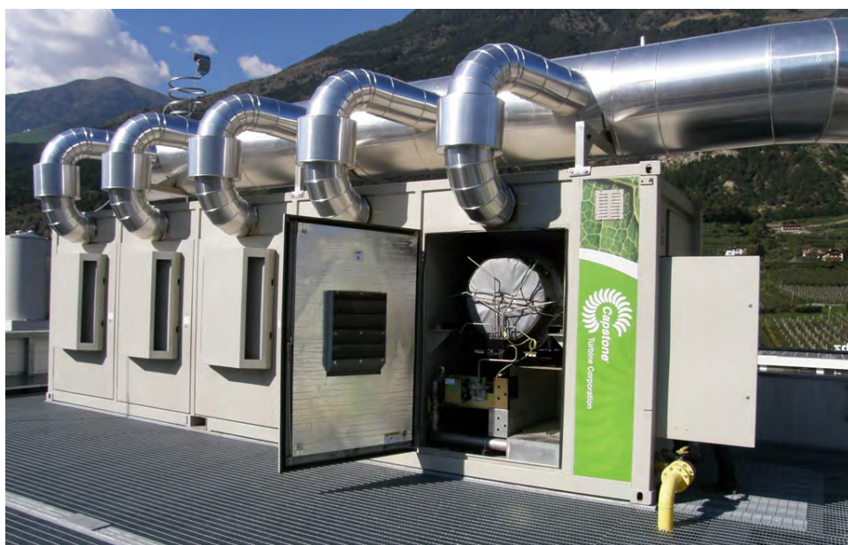
Figure 2-5. Capstone C1000, 1000 kW microturbine package with integrated exhaust manifold
