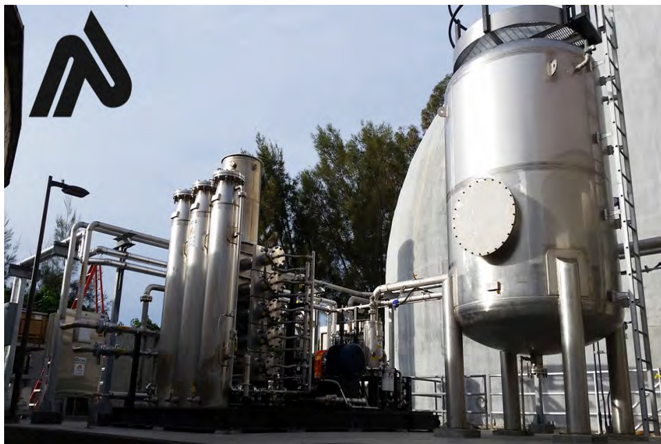
Figure 2-2. Biogas upgrading system at San Mateo WWTP (CA) using Unison's BioCNG system
