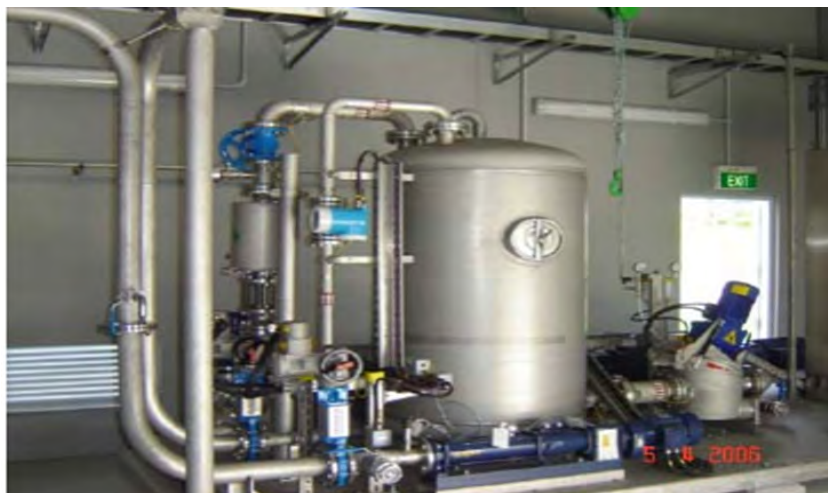
Figure 4-4. Crown™ disintegration system at Rosedale WWTP, North Shore, New Zealand
