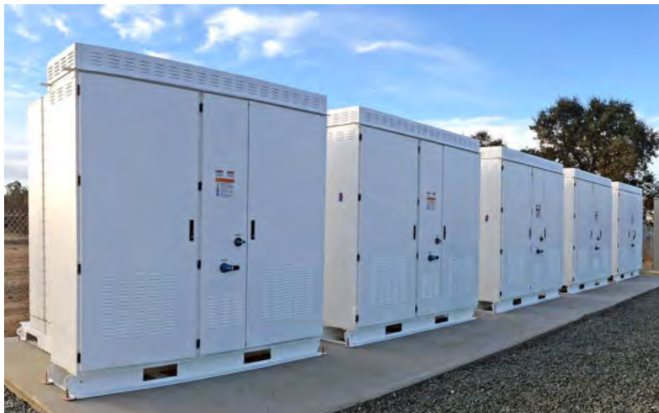
Figure 2-6. Napa Sanitation's Tesla Batteries
