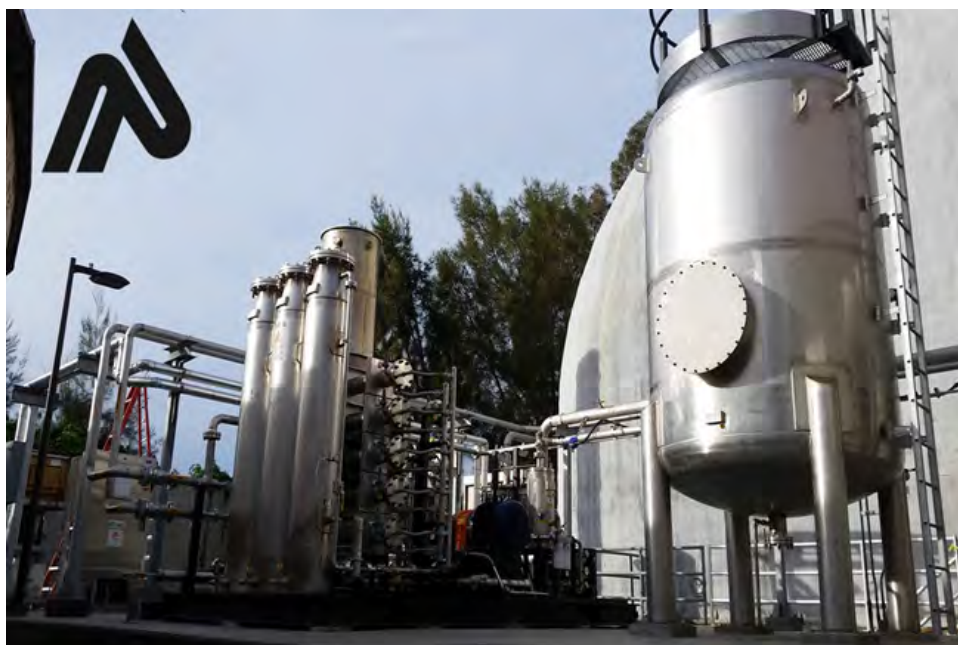
Figure 2-3. Biogas upgrading system at San Mateo WWTP (California) using Unison's BioCNG system, which includes \text{H}_2\text{S} removal, moisture removal, compression, siloxane removal, and membrane separation
