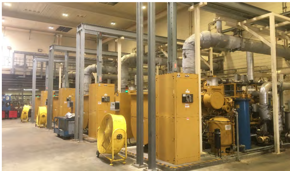
Figure 2-1. Existing 750 kW Caterpillar engines at EWPCF
