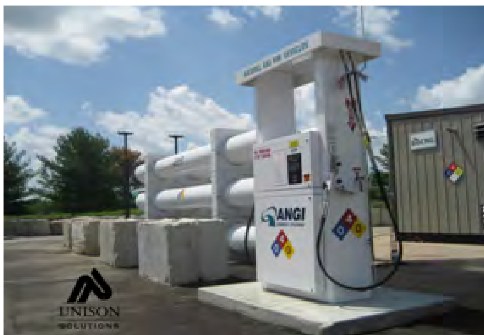
Figure 2-4. Example of ANG1 vehicle fueling equipment, including high pressure storage and fuel dispenser
