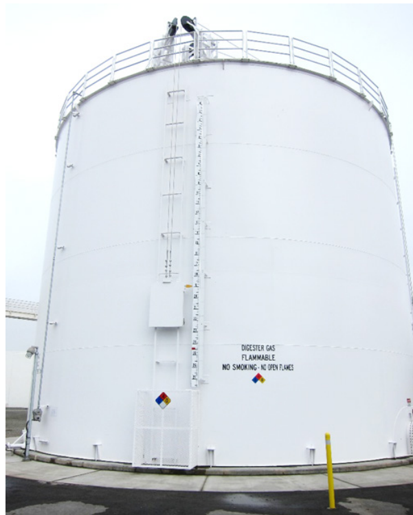
Figure 3-1. Piston-type gas holder installed at SJSCRWF with 50,000 cubic feet of active storage
