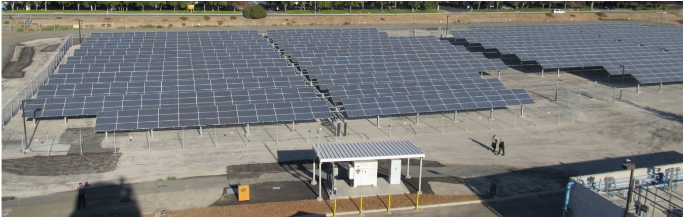
Figure 2-9. Union Sanitary District Irvington Pump Station PV Project included 460 kW of installed solar PV in an emergency overflow basin
