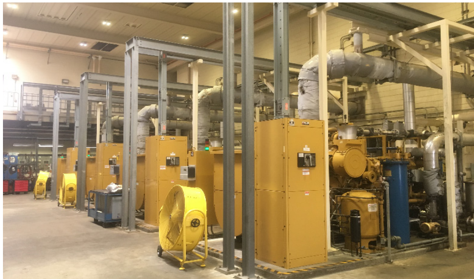
Figure 2-1. Existing 750 kW Caterpillar engines at EWPCF
