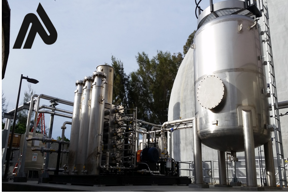
Figure 2-2. Biogas upgrading system at San Mateo WWTP (CA) using Unison’s BioCNG system Includes hydrogen sulfide removal, moisture removal, compression, siloxane removal, and membrane separation.
