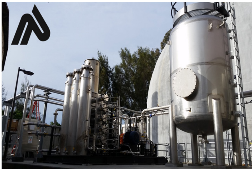
Figure 2-3. Biogas upgrading system at San Mateo WWTP (California) using Unison’s BioCNG system, which includes H 2 S removal, moisture removal, compression, siloxane removal, and membrane separation
