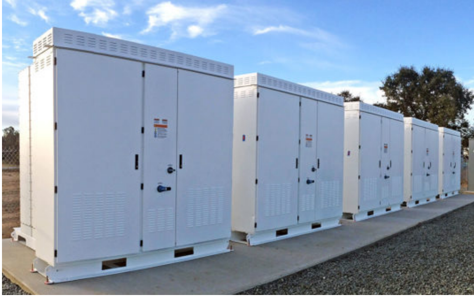
Figure 2-6. Napa Sanitation's Tesla Batteries
