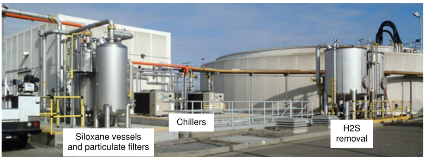
Figure 2-1. Gas conditioning system at the Santa Rosa Laguna Treatment Plant, including H 2 S removal vessels, siloxane removal vessels, and chillers
