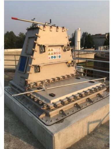
UTS Mixer Access Hatch
