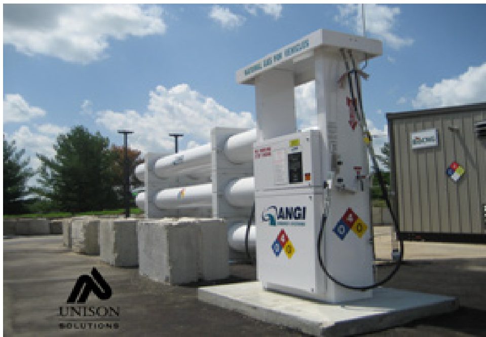
Figure 2-4. Example of ANGI vehicle fueling equipment, including high pressure storage and fuel dispenser
