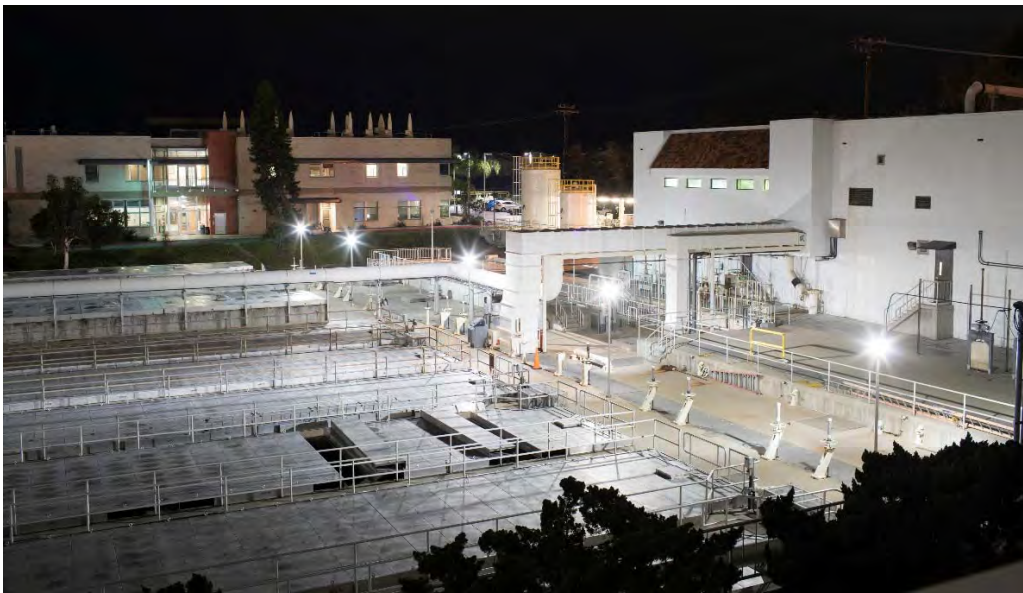
Primary Treatment (front) and the Grit & Screenings Handling Facility (right)
