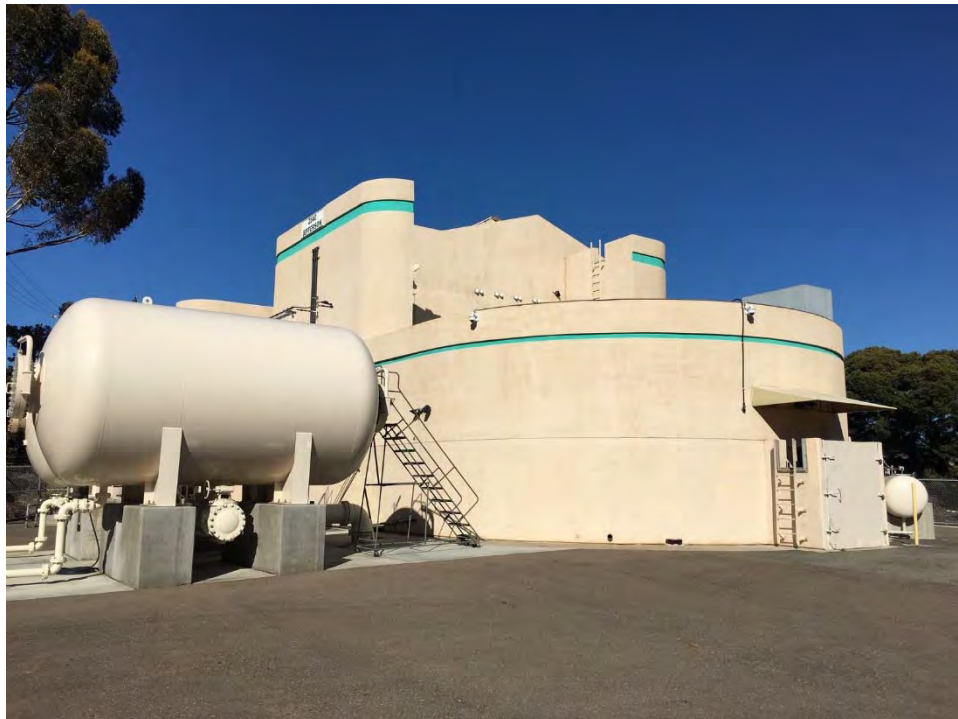
Buena Vista Pump Station
