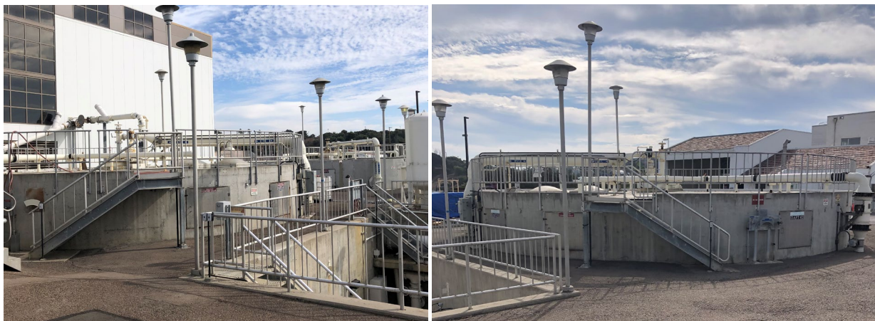
Figure 1-9. Dissolved Air Flotation Thickeners
