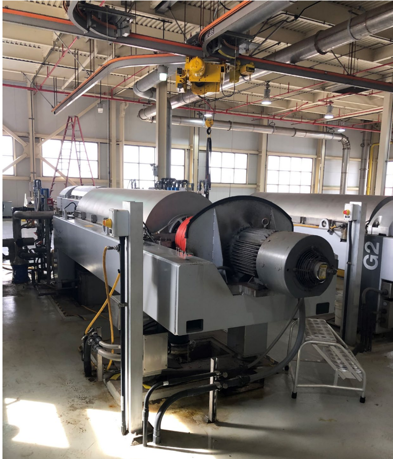
Figure 1-14. Three Existing Centrifuges
