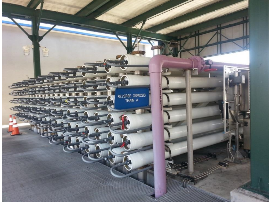
Figure 4-4: City of Los Angeles Terminal Island AWPF RO Train
