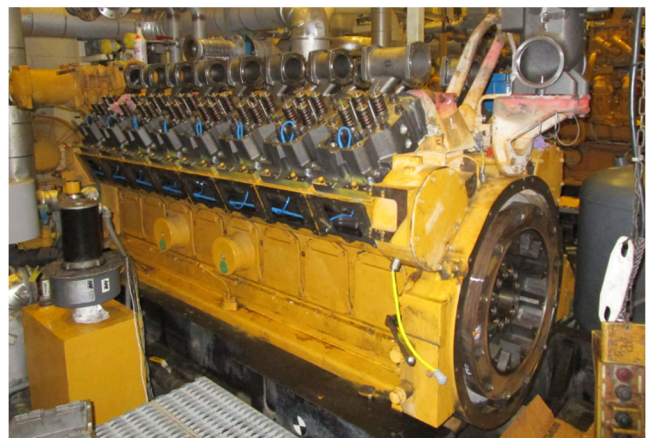
Overhaul on a 1,000 horsepower engine
