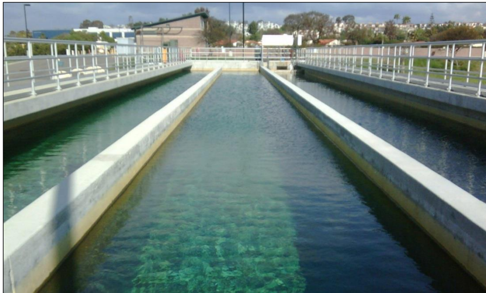
Carlsbad Water Recycling Facility
