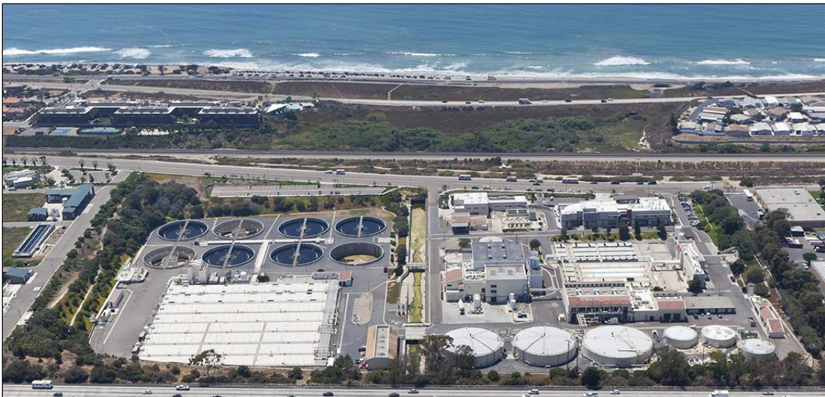
Encina Pollution Control Facility
