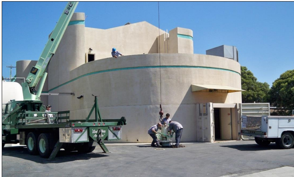
Buena Vista Pump Station
