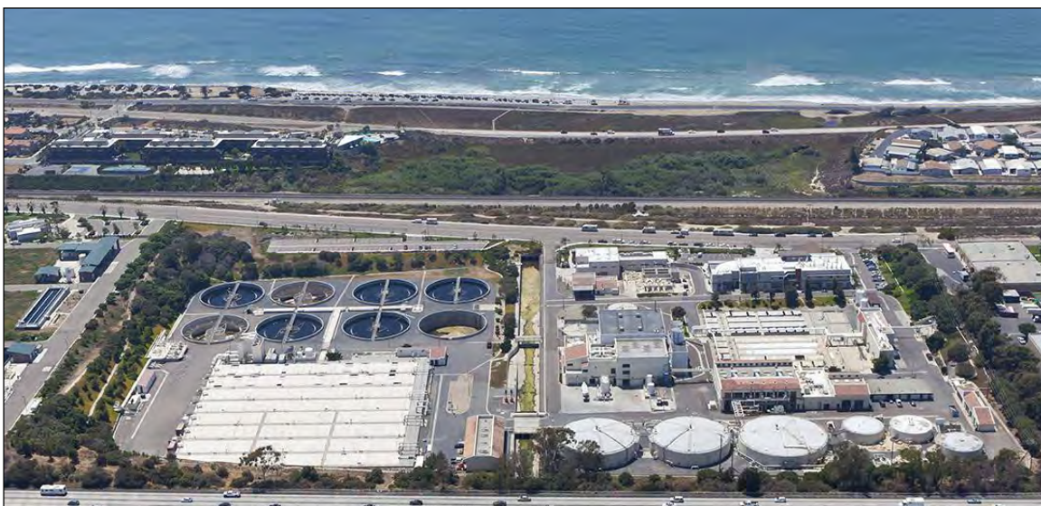
Encina Pollution Control Facility
