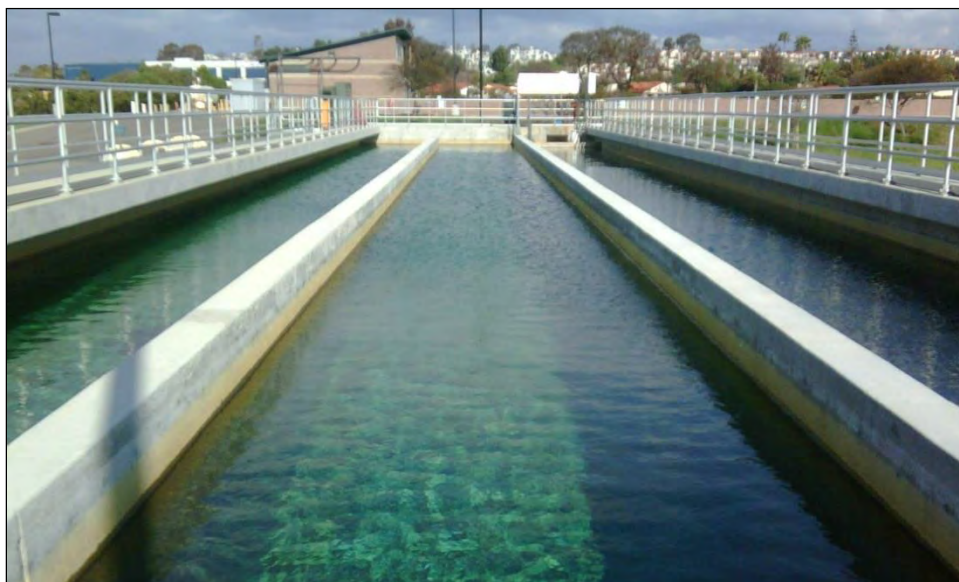
Carlsbad Water Recycling Facility
