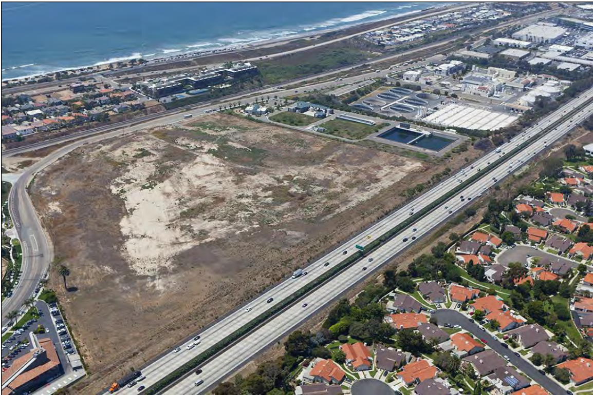
Encina Water Pollution Control Facility
