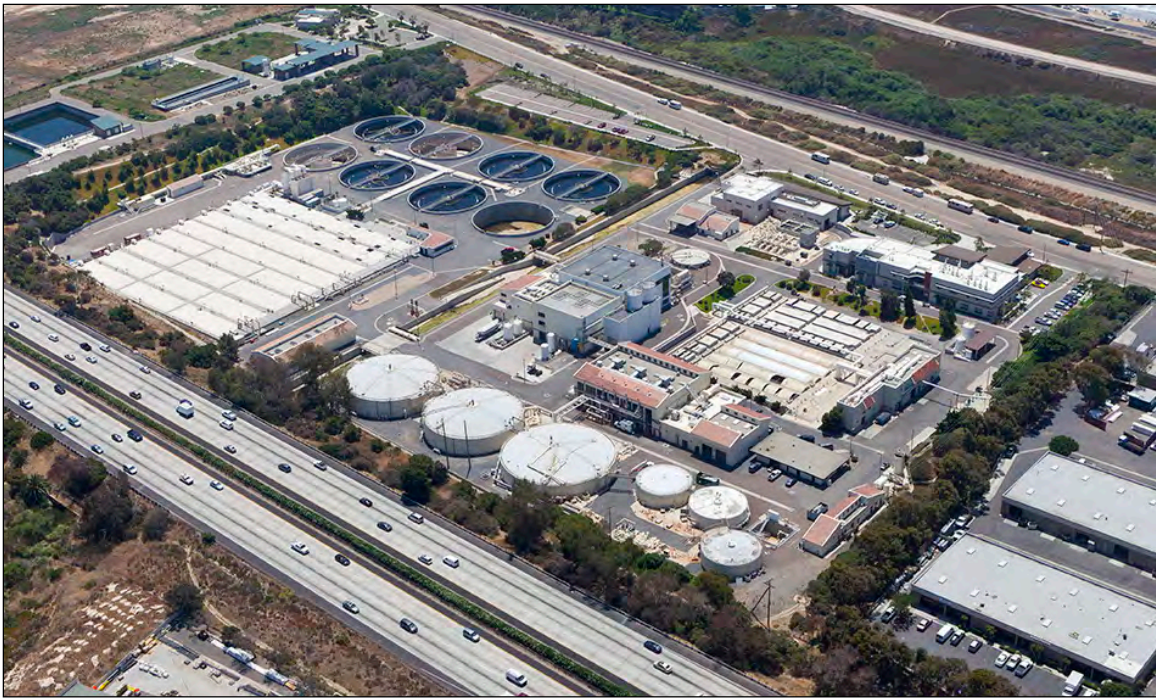
Encina Water Pollution Control Facility
