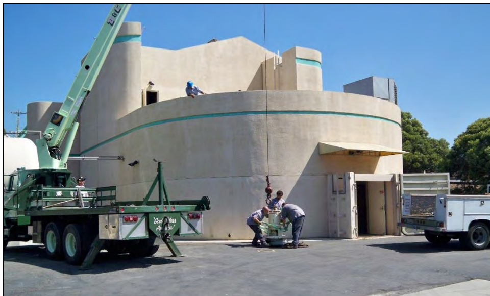
Buena Vista Pump Station
