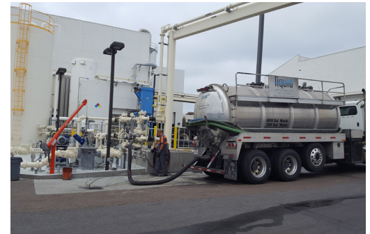
Restaurant grease generates additional biogas to offset natural gas use.
