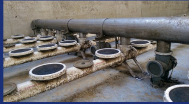
Old piping and diffusers
